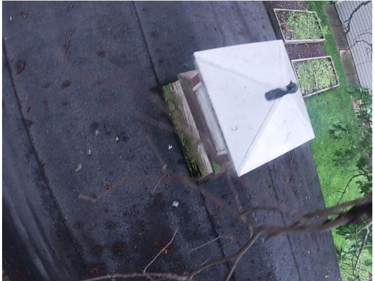
Shed. Picture of roof of shed.
