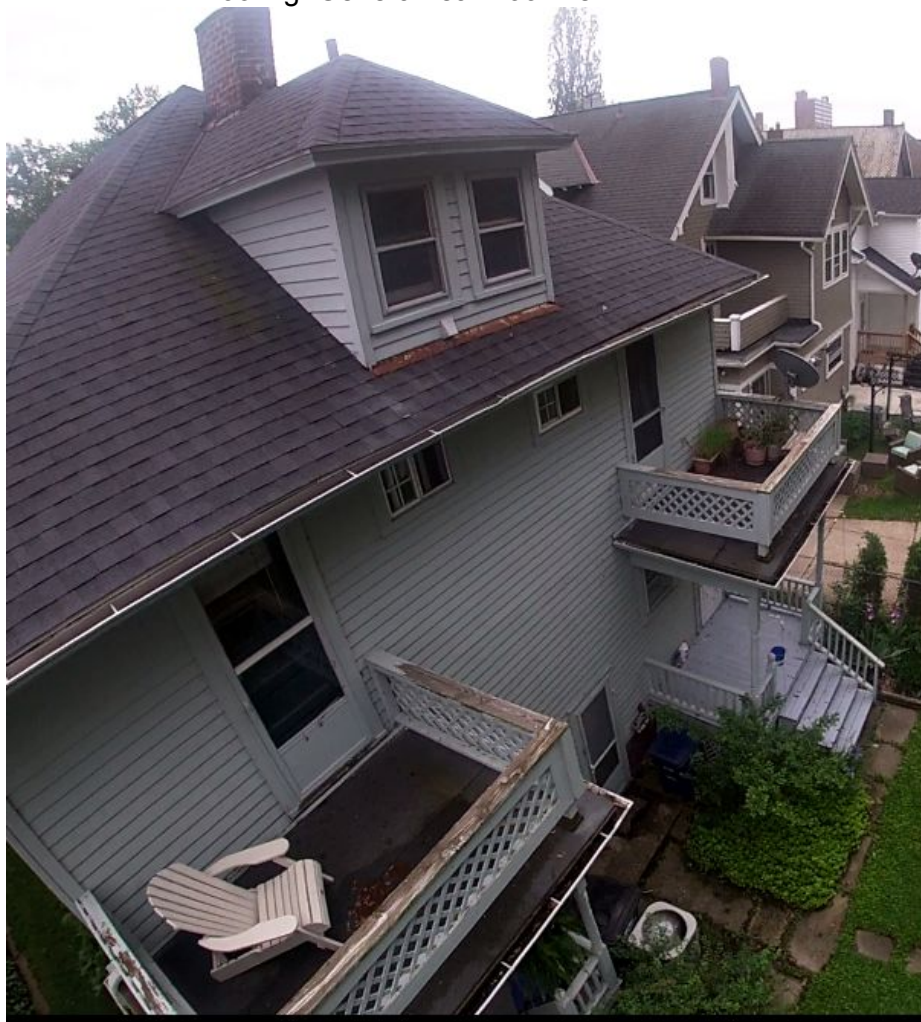
Roofing. General rear roof view.
